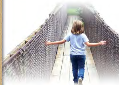
Whitewater Gorge Swinging Bridge
